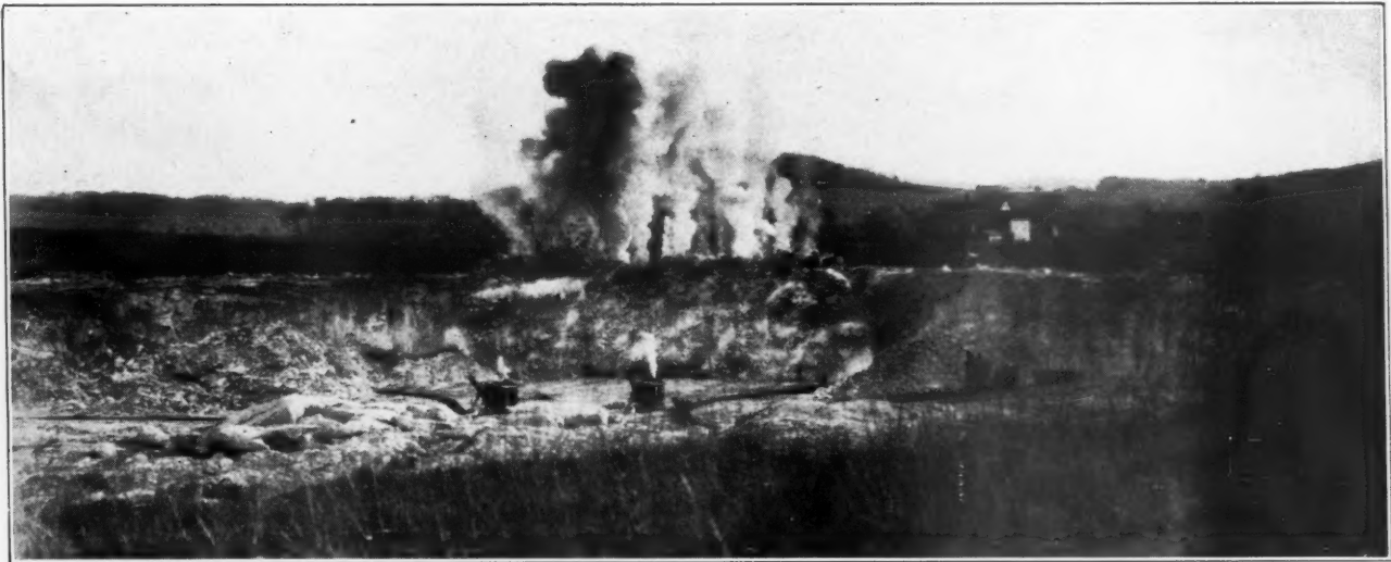
Blast which Released 50,000 Tons of Stone.
